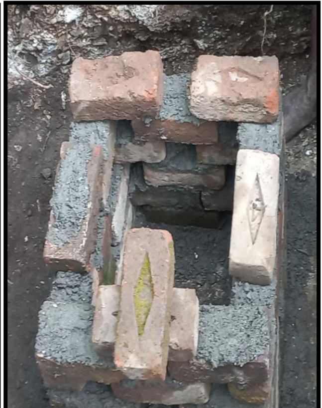
Soak Pits at Beside of Chemistry Laboratory
